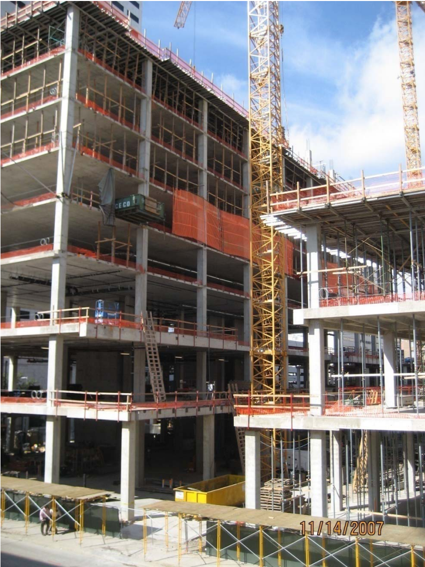
LEFT PHOTO – BLOCK 273 VIEW FROM BLOCK 274 ROOF.
