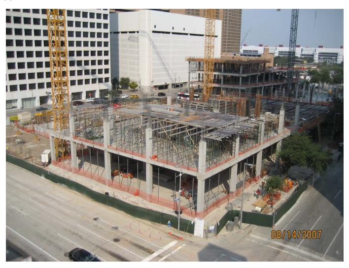
BLOCK 272 - CONCRETE SLAB ON GRADE FOR 272 SOUTH HAS BEEN POURED.
