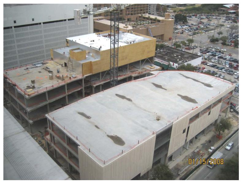
BLOCK 273 - OFFICE TOWER ROOF AND PENTHOUSE CONCRETE WORK "TOPPED OUT".
