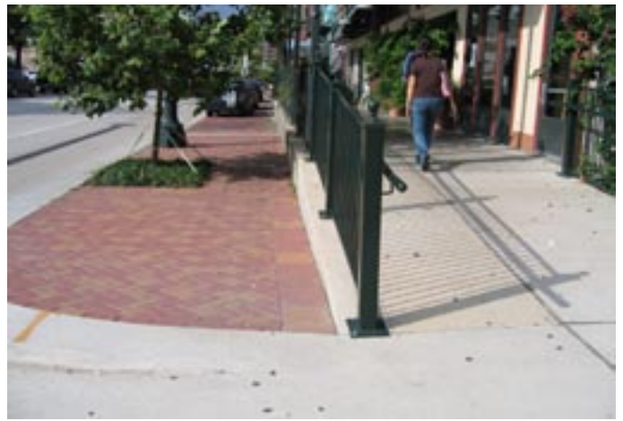
The east sidewalk across the street could be reconfigured to be more gracefully accessible.
